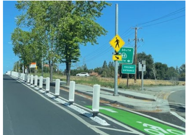
Figure 7: Class IV bikeway with Qwick Kurb at SR 82 and SR 87
