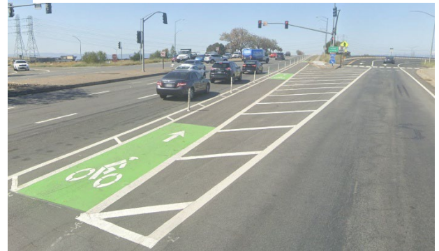
Figure 6 Partially Separated Floating Bike Lane at an Interchange in Fremont, CA
