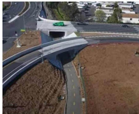
Class I (Multi Use Path) Bike/ped undercrossing at an on ramp/ of ramp at US 101/Blossom Hill Rd
