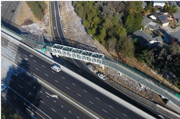
Class I (Multi Use Path) Bike/ped overcrossing at an on ramp at US 101/Blossom Hill Rd
