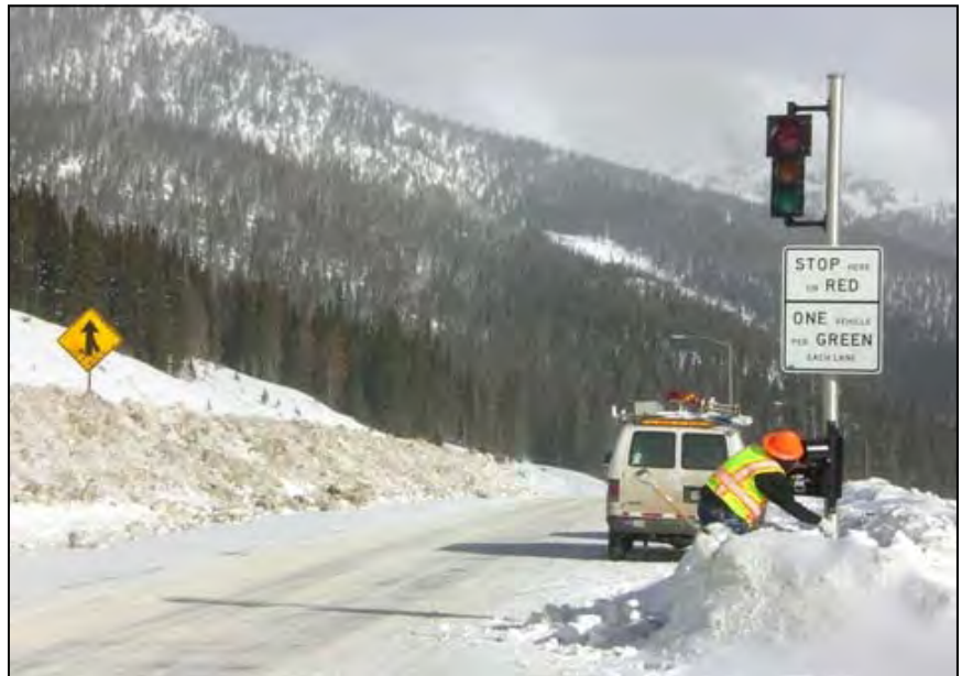
Steve Smith, CDOT Region 1, performs maintenance on the east-bound I-70 & Loveland Pass ramp meter.
