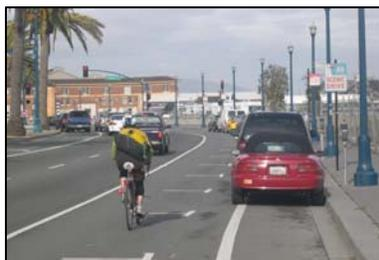
**Contra-Flow Bike Lane** – East Conservatory Drive in Golden Gate Park used to be a one-way road before it was converted to two-way for cyclists. Prior to the conversion cyclists were riding illegally on pedestrian paths or against traffic or taking the long way around. The street now functions as a two-way street with cars not allowed in one direction.
