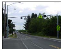
Photograph of crosswalk flasher installation.
