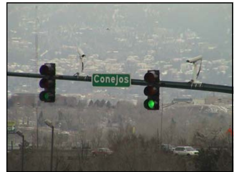
Two cameras mounted on same mast arm
