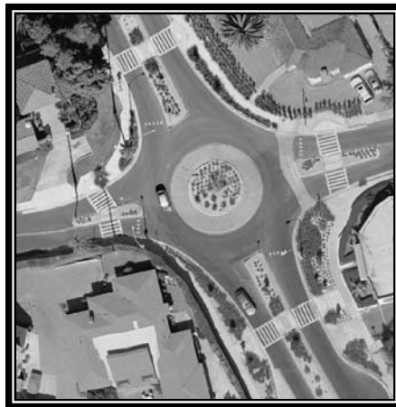
Aerial photo of La Jolla Blvd/Camino de La Costa, after the improvement.
