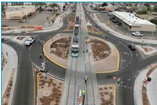
Figure 6: Gilbert Road Extension Roundabout
