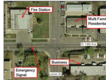
Existing conditions at the Intersection
