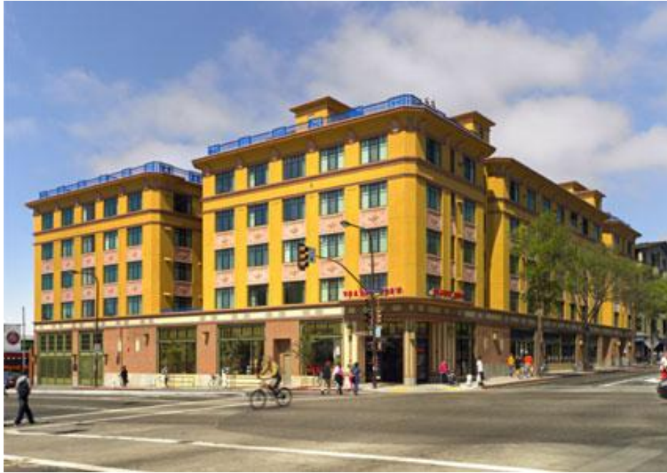
Figure 1: Exterior Photo of New Californian Apartments
