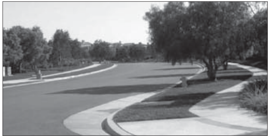
Figure 4. Chambord Road before restriping.
