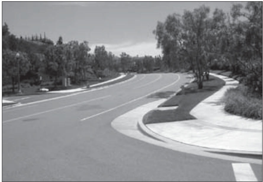
Figure 1. Typical traffic calming striping.
