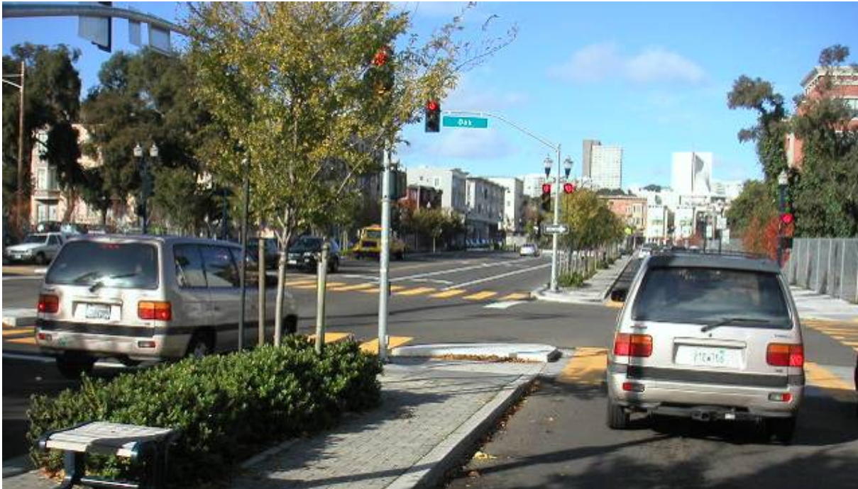
FIGURE 5: OAK STREET AT OCTAVIA BOULEVARD. VEHICLE ON THE RIGHT CAN PROCEED STRAIGHT AFTER STOP WHILE THE VEHICLE ON LEFT MAKES A RIGHT TURN ON GREEN LIGHT
